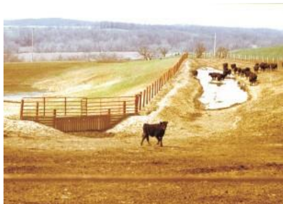
Solids settling structure with slotted gate.
